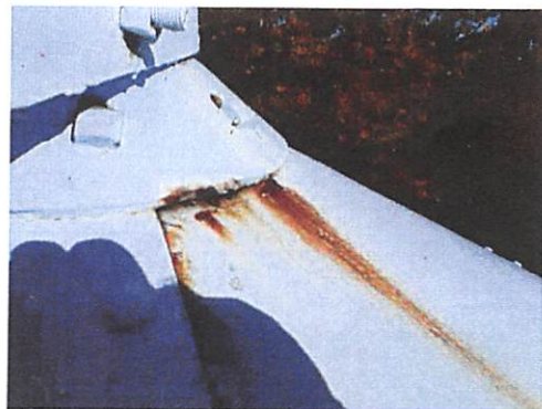
Roof exterior: showing finial ball connection to roof to be visually acceptable at least as viewed from the exterior of the tank.
